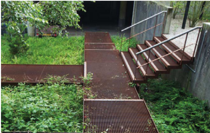
Farum Midtpunkt. Ramboll Architecture and Urban Development. Seeland, Danemark
